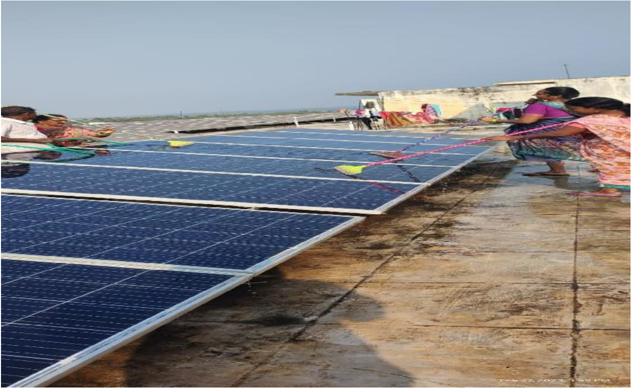
Solar Panel Cleaning
